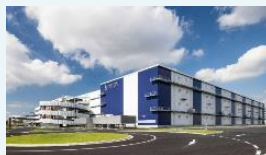
LOGIPOINT Nagoya Completed in Jul. 2023
