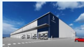
Yatabe Logistics Center Scheduled completion in Feb. 2025
