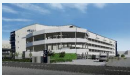
Logiport Amagasaki 2 Scheduled completion in Jul. 2025
