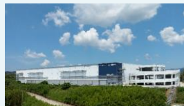
LOGIPOINT Fukuoka Kasuya Completed in Aug. 2024
