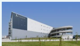
LOGIPOINT Tama Mizuho Completed in Jun. 2024
