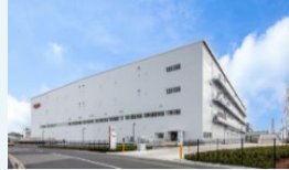
Matsudo Logistics Center Completed in Jan. 2022
