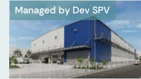
Matsudo Project Scheduled completion in Sep. 2024
