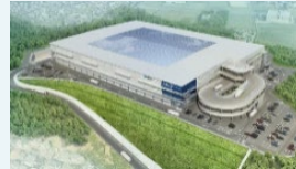
LOGIPOINT Fukuoka Kasuya Scheduled completion in Aug. 2024
