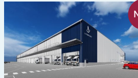
Yatabe Logistics Center Scheduled completion in Feb. 2025
