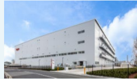
Matsudo Logistics Center Completed in Jan. 2022
