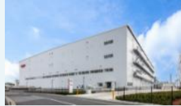
Matsudo Logistics Center Completed in Jan. 2022
