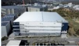
LOGIPORT Kobe Nishi Completed in Nov. 2021
