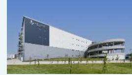
LOGIPORT Tama Mizuho Completed in Jun. 2024
