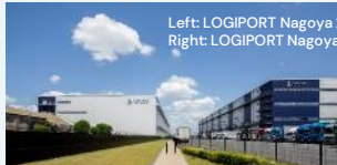
Left: LOGIPORT Nagoya 2 Right: LOGIPORT Nagoya Completed in Jun. 2025
